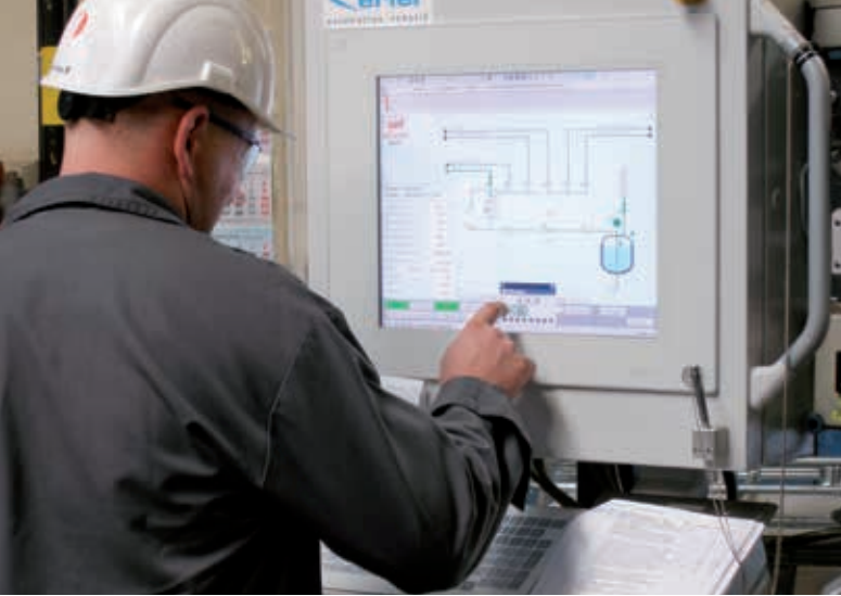
In addition to the APROL process control system, CHT is also adopting B&R's X20 control system. The new solution includes a total of 46 Power Panel HMI units from along with countless other control and I/O modules B&R.
